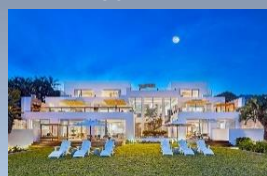
THE WHITE HOUSE BOUTIQUE VILLA
